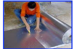
**Step 3:** Starting from the edge, secure CoolMax to the existing frame, (leave 10 to 15cm (4 to 6 inches) of extra "tail" (figure 3a) to be cut later, when work is completed). Move along or across the frame and fix CoolMax with staple pins (if frame made of wood) or self tapping screws (if frame made of metal) see 3b illustration. Fix CoolMax to each frame line (trusses). Make sure to stretch the CoolMax shreds to avoid sagging.
