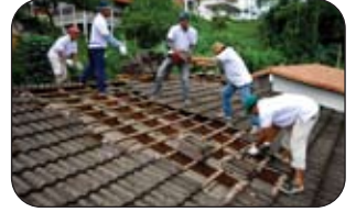
4 | Dismantle existing old roof tiles, portion by portion.
