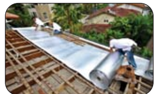
8 | Lay COOLMAX insulation foil.
