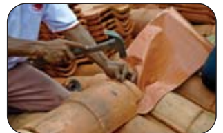
12 | Install ridge tree and ridges using Terreal Dry Fix.
