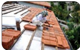
11 | Lay new Terreal roof tiles.
