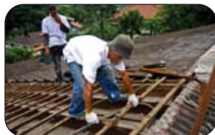
7 | Remove batten and inspect conditions of each batten.
