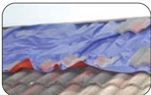
5 | In case of raining, exposed roof will be covered with canvas.
