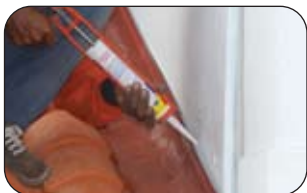
13 | Install wall flashing using Terreal Dry Flash.
