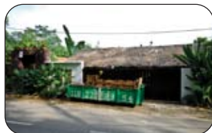
15 | Gathering, clearing of rubbish and debris.
