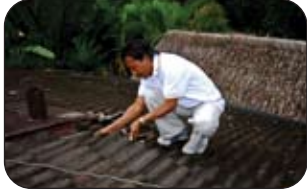
1 | Roof inspection by Terreal Certified Installation Partner
