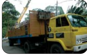
3 | Arrival of roofing materials, equipment and necessary transport.
