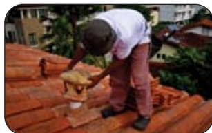
14 | Install socket and lantern for ventilation outlet.
