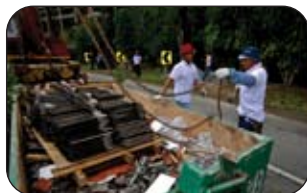
6 | Dispose old tiles into a disposal bin.
