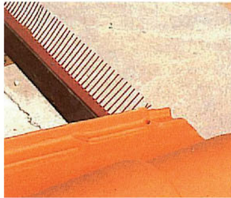
Nail the bird stop on top of the fascia board.
