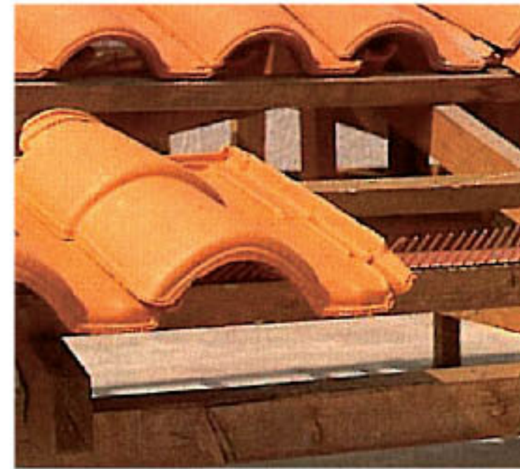
Nail the bird stop on the eave batten.
