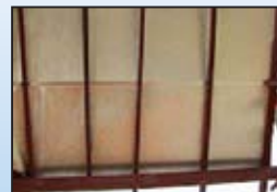
Step 7 View from roof underneath.
