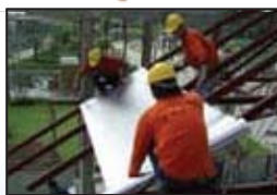
Step 2 Starting from trusses edge, lay CoolMax™ across the purlins.
